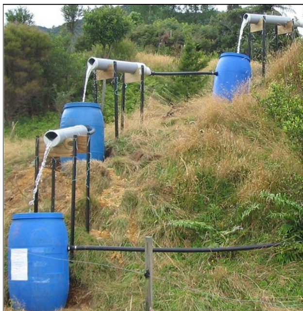
Fig. 6 First three V-notch weirs and barrels in the oxygenation cascade
